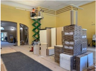
Installing Library Millwork
