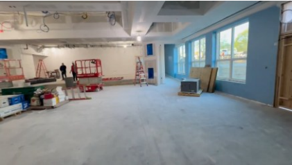
Drywall Finishing Cafetorium Stage
