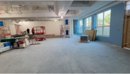
Drywall Finishing Cafetorium Stage
