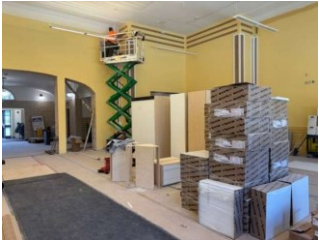
Installing Library Millwork
