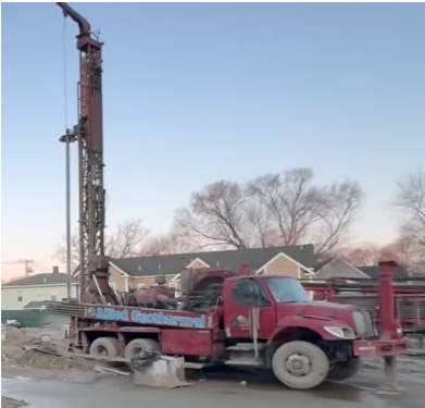
Geothermal Well Drilling
