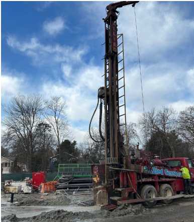
Geothermal Well Drilling
