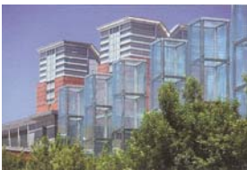
Parcel 7 Mixed-Use Vent Building, Boston
