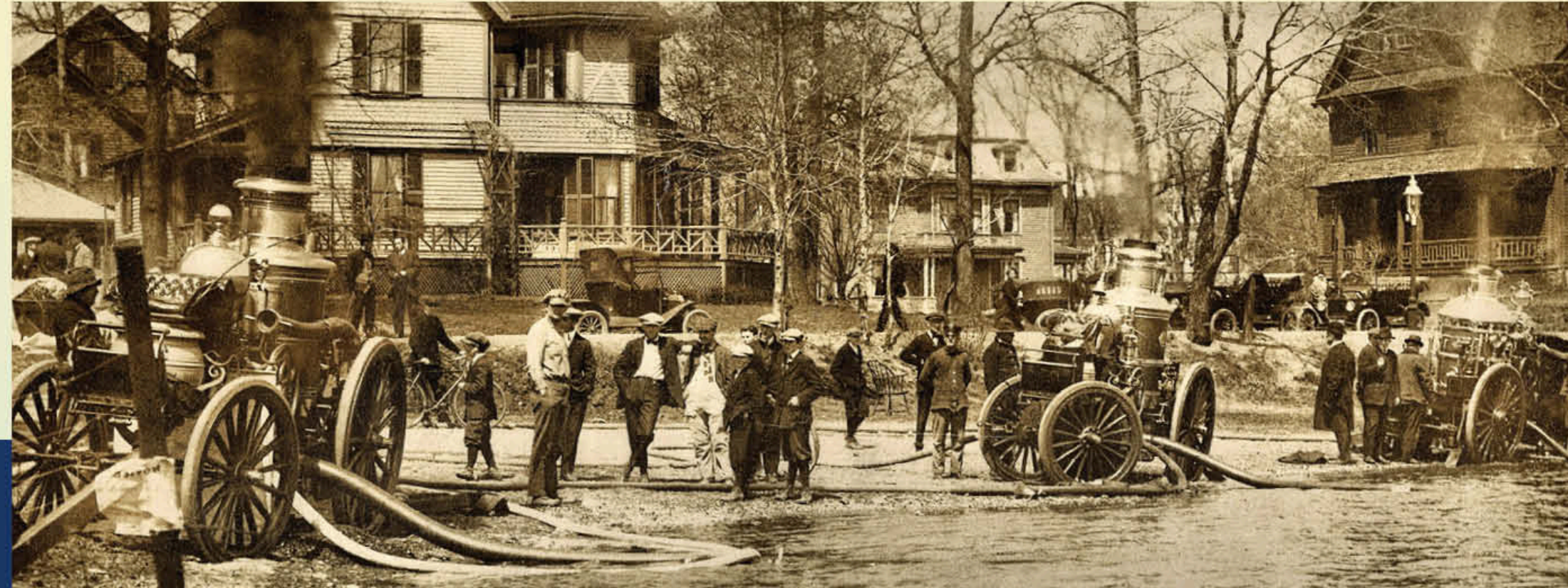
The aftermath of the 1915 Crystal Lake Ice House fire. Norwood Avenue is in the background.
