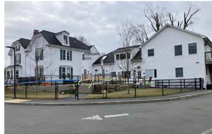
VIEW FROM REAR PARKING AREA
