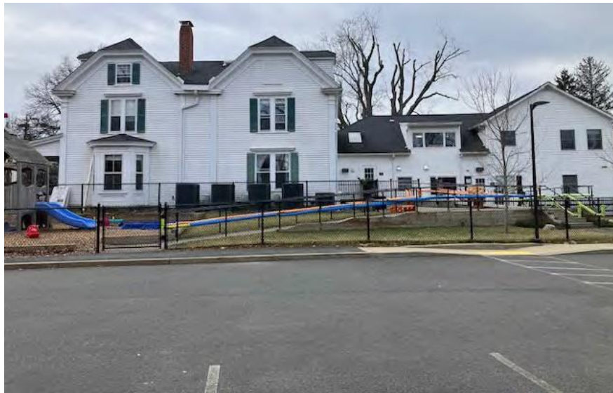
VIEW FROM EAST PARKING AREA
