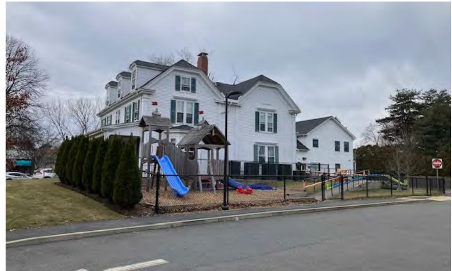
VIEW FROM EAST PARKING ENTRANCE
