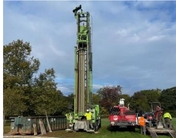
Countryside test geothermal well drilling
