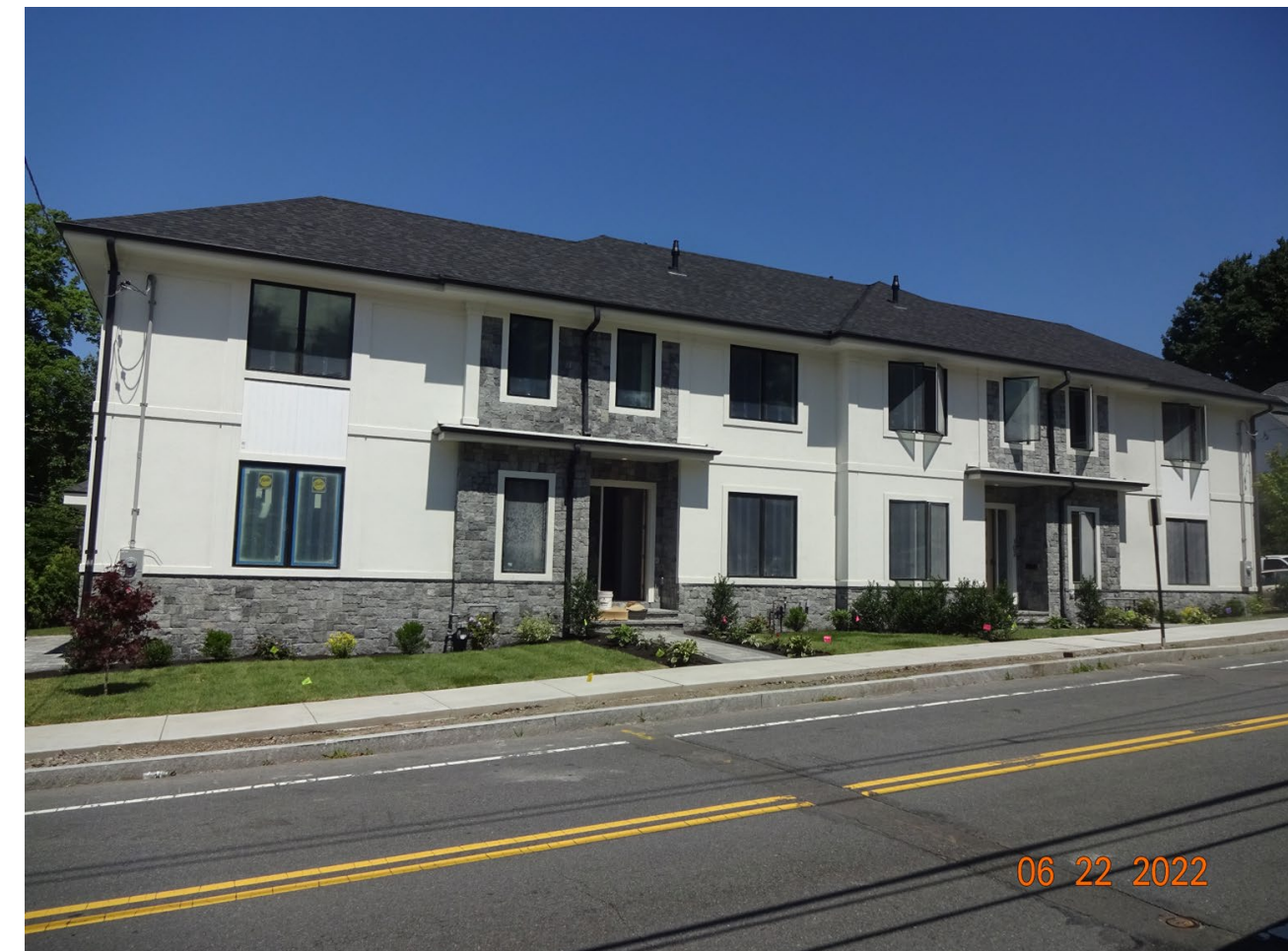
100-102 Langley Rd: 96' Facade
