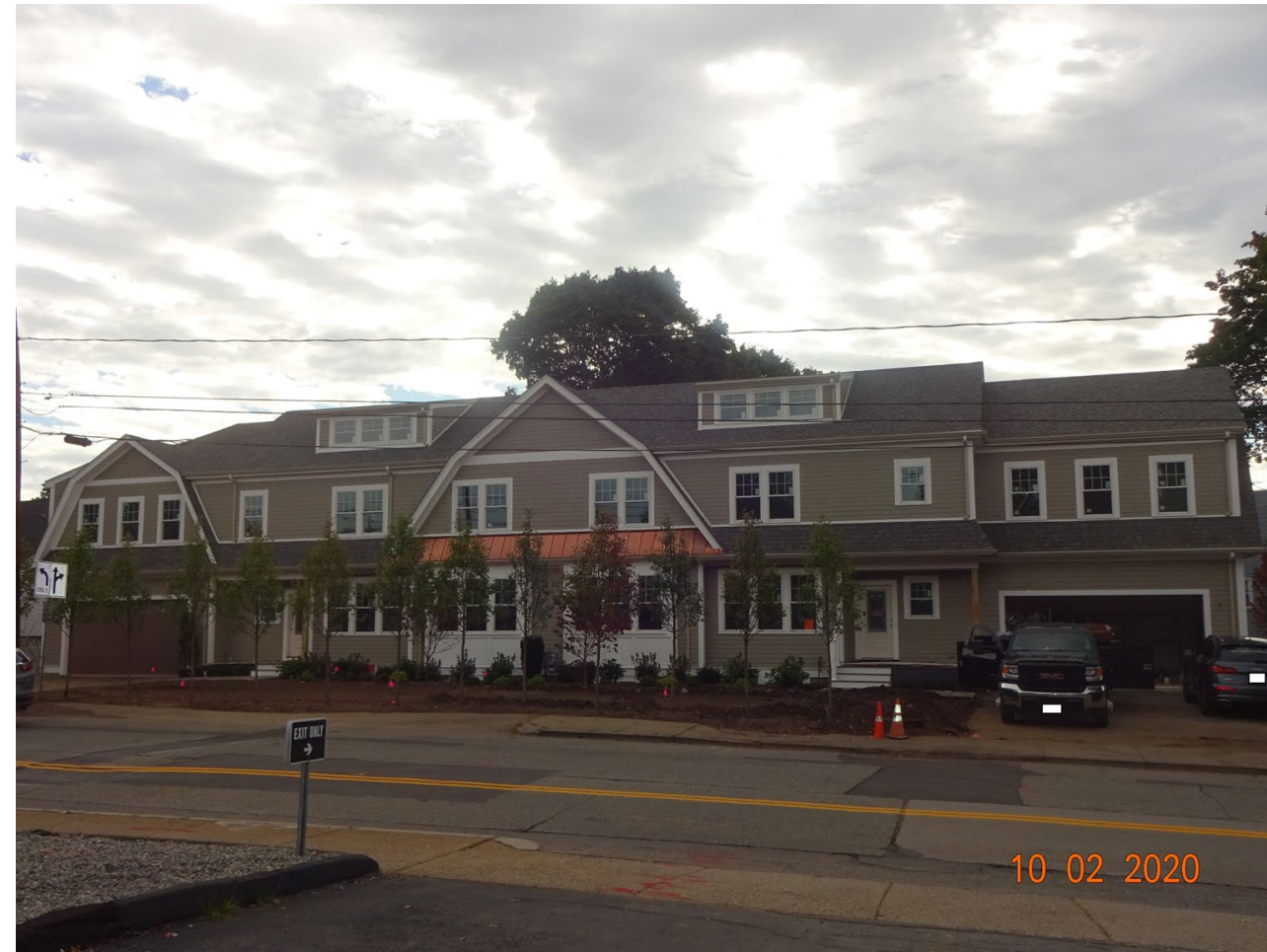
1650-1652 Centre St: 121' Facade
